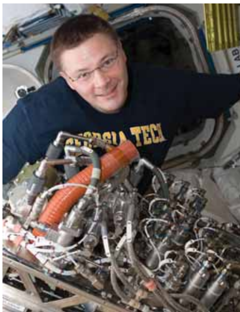
In the Tranquility node aboard the International Space Station, NASA Astronaut Doug Wheelock, Expedition 25 commander, works to install the new Sabatier. Photo Credit: NASA
