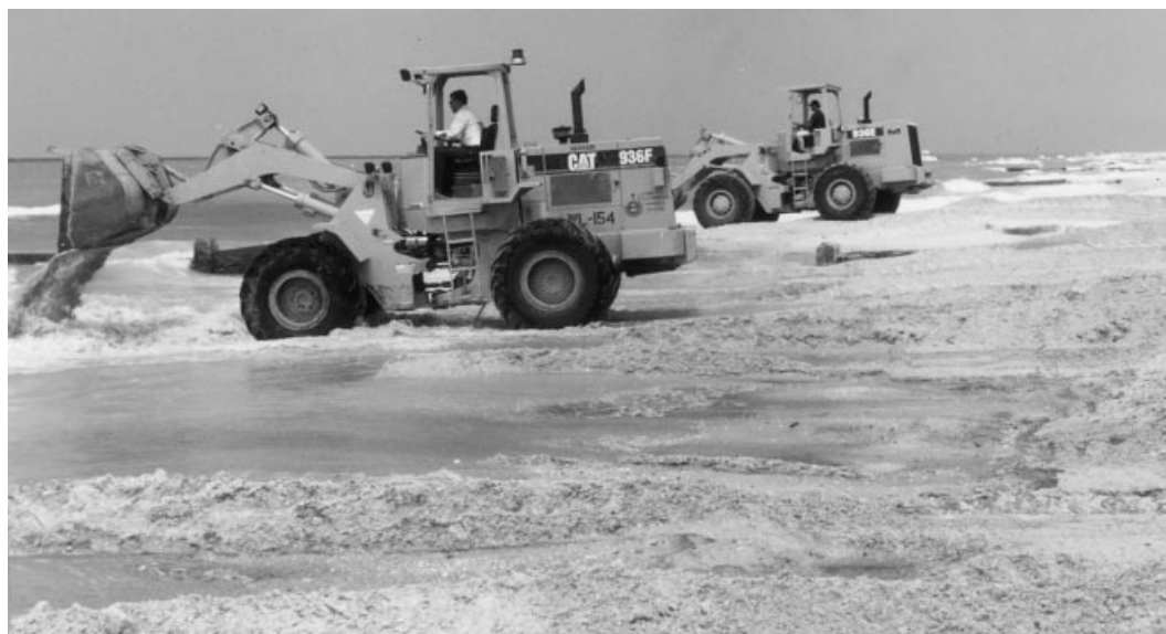
Fig. 3 Photograph of sediment relocation into the surf zone on 21 August 1993: Treasure Island, Florida.
